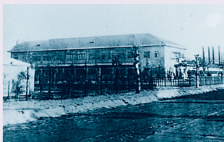
New laboratory of Okayama Plant
